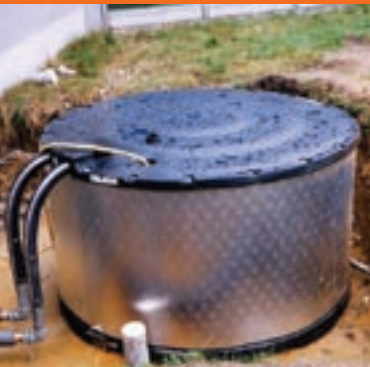
Fig. 2 Ice storage, 170 kWh capacity, IWG Gladbeck
